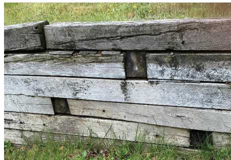
Treated wood retaining wall
